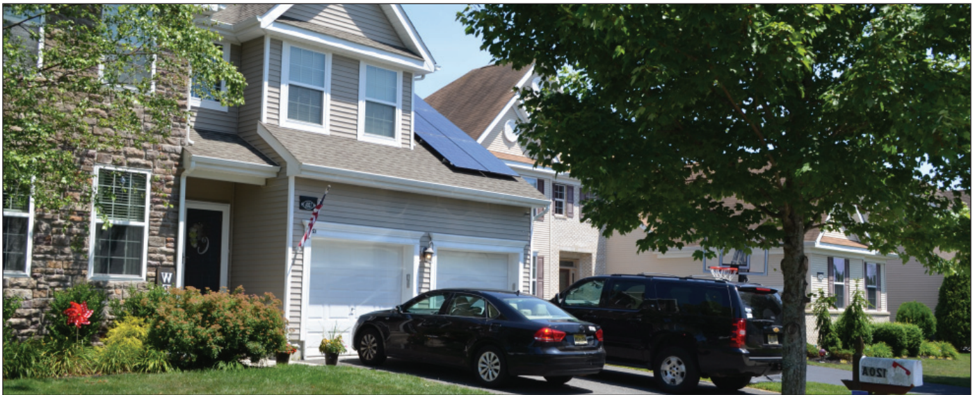
The Crystal Lakes development in Egg Harbor Township, Atlantic County, is an example of a development that was constructed with Pinelands Development Credits.
